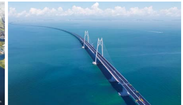
Hong Kong - Zhuhai - Macau Bridge
